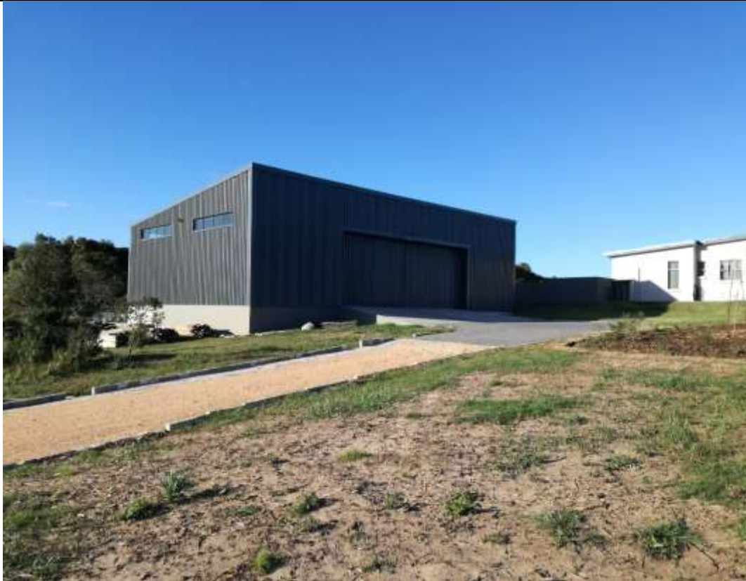
View of access road leading toward shed
